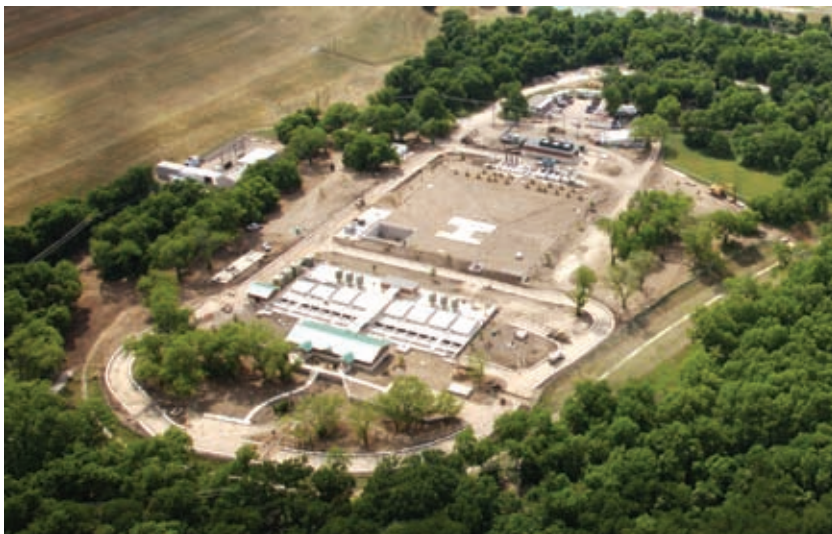
Aerial view of the DAF plant site - May 2010
